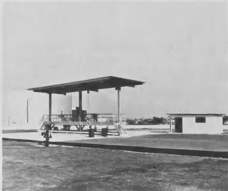
The new main facilities where jet fuel, gasoil, motor gasolines and aviation gasoline can be loaded safely and efficiently can be seen here with a small office for the loading rack operator.
